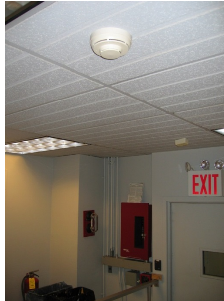
Chemetron FM-200 with Notifier Control Panel and Fike Selector Switch
