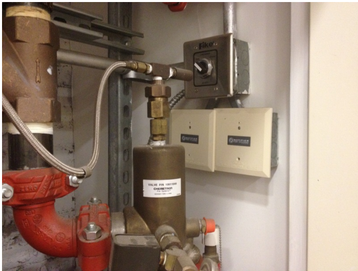
Chemetron FM-200 with Notifier Control Panel and Fike Selector Switch
