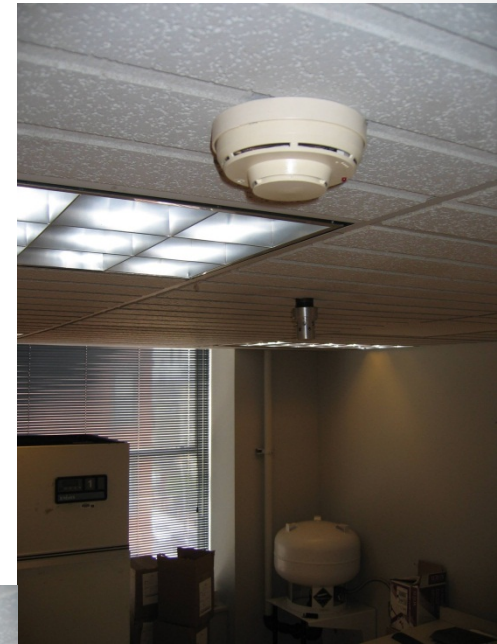
Fike FM-200 with Kidde Control Panel and Pyrotronics Smoke Detectors
